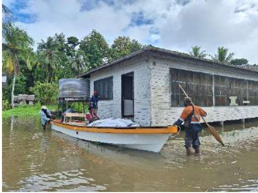
Photo 1: Health facility visit to Marienberg HC. Dispensary submerged under water.
